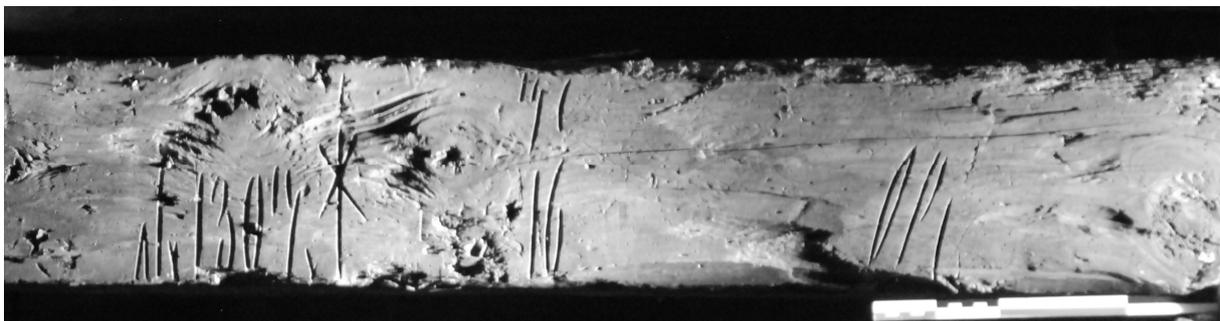
Figure 5. Merchant’s timber marks, Godin Factory, Brussels. © SPRB
