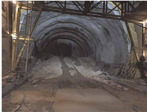
**Figure 18.** Tunnel inner lining section (a) tunnel section (b) application in site.
