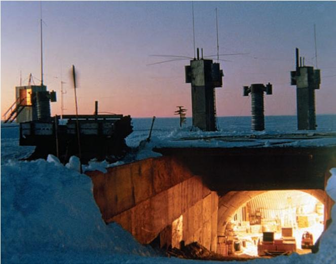
Fig. 8: Ramp of the Georg von Neumayer Station (GvN) as the entrance for vehicles into the cross tube and workshop (AWI).
