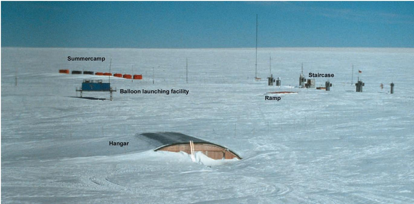
**Fig. 6:** Area view of Georg von Neumayer Station (GvN) in 1989. In front the aircraft hangar almost completely covered by snow. Entrance towers, exhaust pipes and antenna domes in the right centre mark the position of the GvN structure beneath the snow. Behind the balloon-launching container (centre left) of the meteorological observatory the red emergency huts are visible in the background (AWI).
