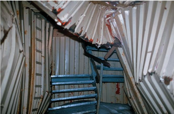
Fig. 9: Georg von Neumayer Station (GvN) in 2000. Eight years after abandonment of the station the staircase shows strong demolition by ice pressure.
