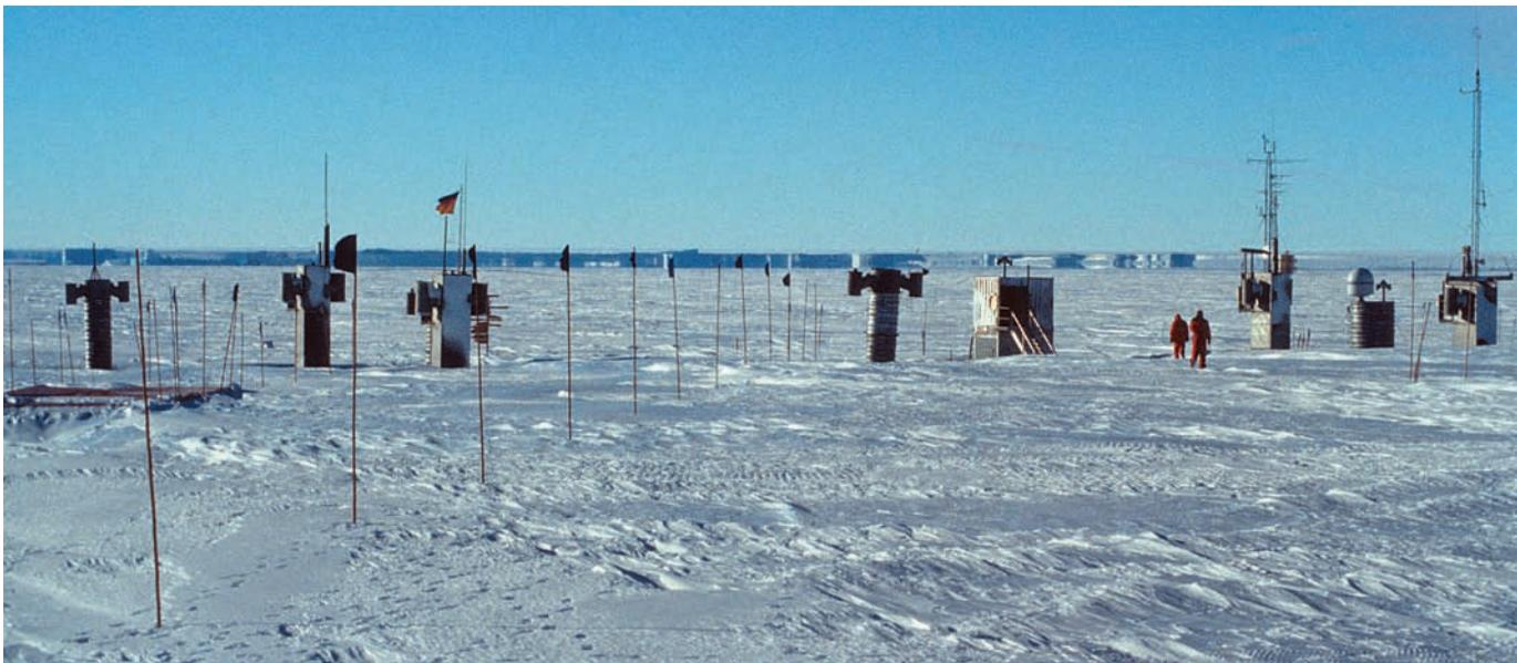
**Fig. 7:** Georg von Neumayer Station (GvN) in 1989. Staircases, ventilation shafts and antennas roughly mark the position of the station beneath the snow surface. The four emergency exit towers indicate the ends of the tubes.
