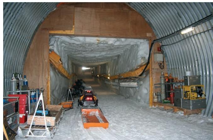
**Fig. 16:** View from the cross tube through the ice tunnel between the vehicle garage and the cross tube of Neumayer Station II (NM-II) in 2005. The original roof construction can be recognized in the walls of the ice tunnel indicating the roof level of the tunnel at the time of construction (AWI).
