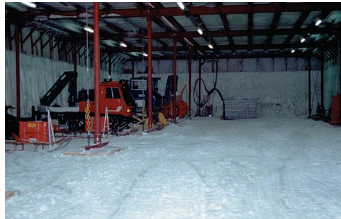
**Fig. 15:** View into the vehicle garage of Neumayer Station II (NM-II) in 1999. The garage is built into the firm with a new type of roof construction, which is regularly corrected according to the snow accumulation and surface.
