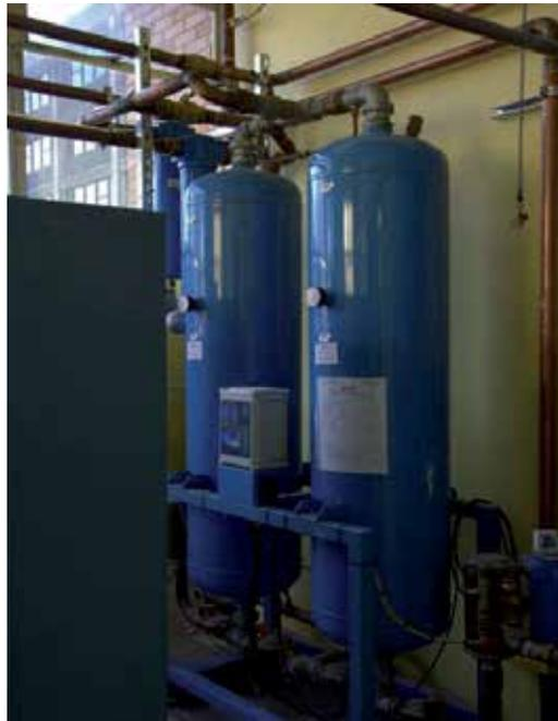
**Figure 4.** Air Drier System
